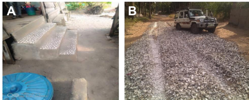
Figure 4: Use of shellfish product including (a) the use of cockle shells for tiling steps and (b) oyster shell used in feeder road construction and maintenance by coastal communities.
